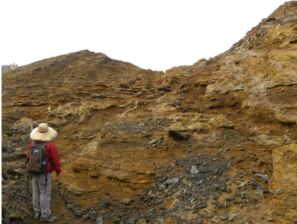
Figure 3. Studying a destabilized zone in a tailings impoundment located at La Unión (Murcia).
